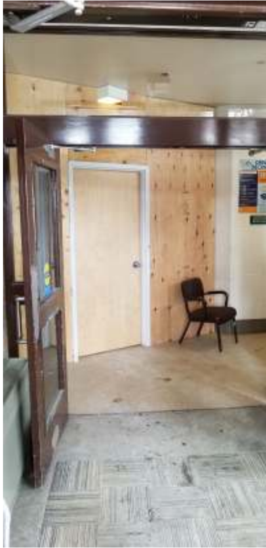
Main Entry - Now
