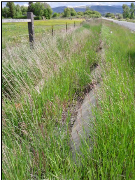
Photo 4.4: Concrete irrigation channel at MP 0.67.
