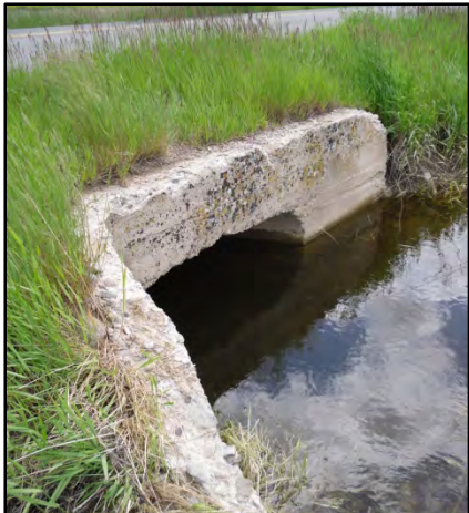
Photo 4.2: Existing drainage structure at MP 0.78.
