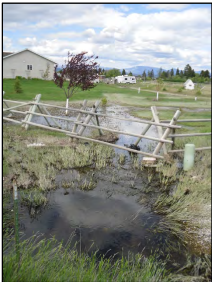
Photo 4.3: Shallow drainage channel downstream of existing cross drain at MP 1.47.
