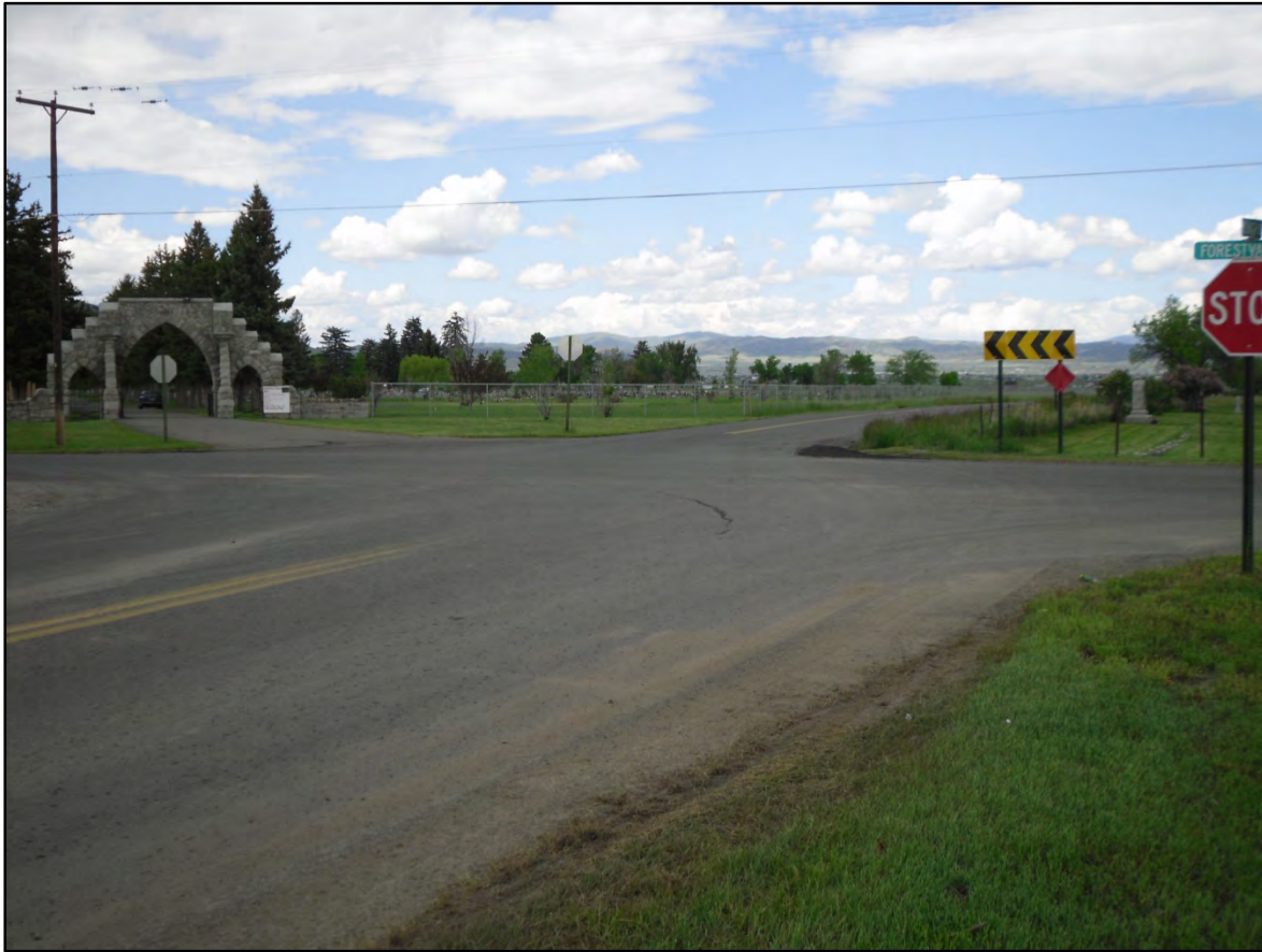
Photo 3.1: Skewed intersection alignment at Forestvale Road.
