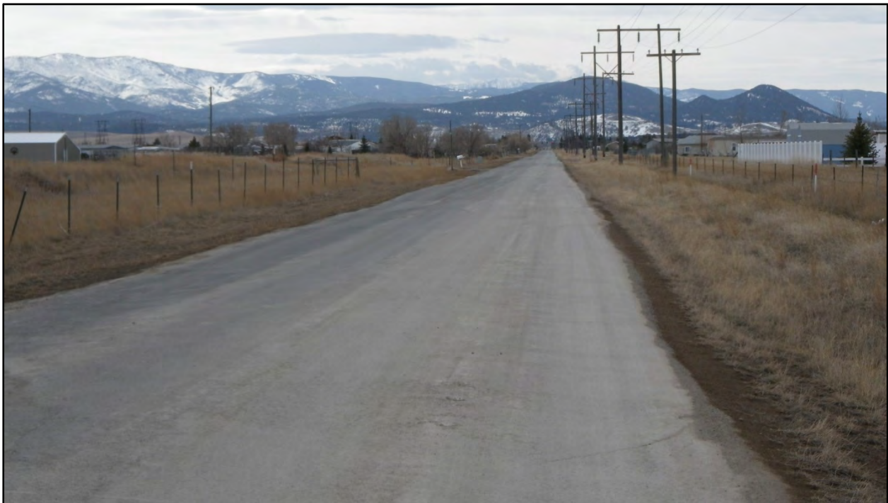
Photo 3.2: Existing Typical Section E.2 looking south.
