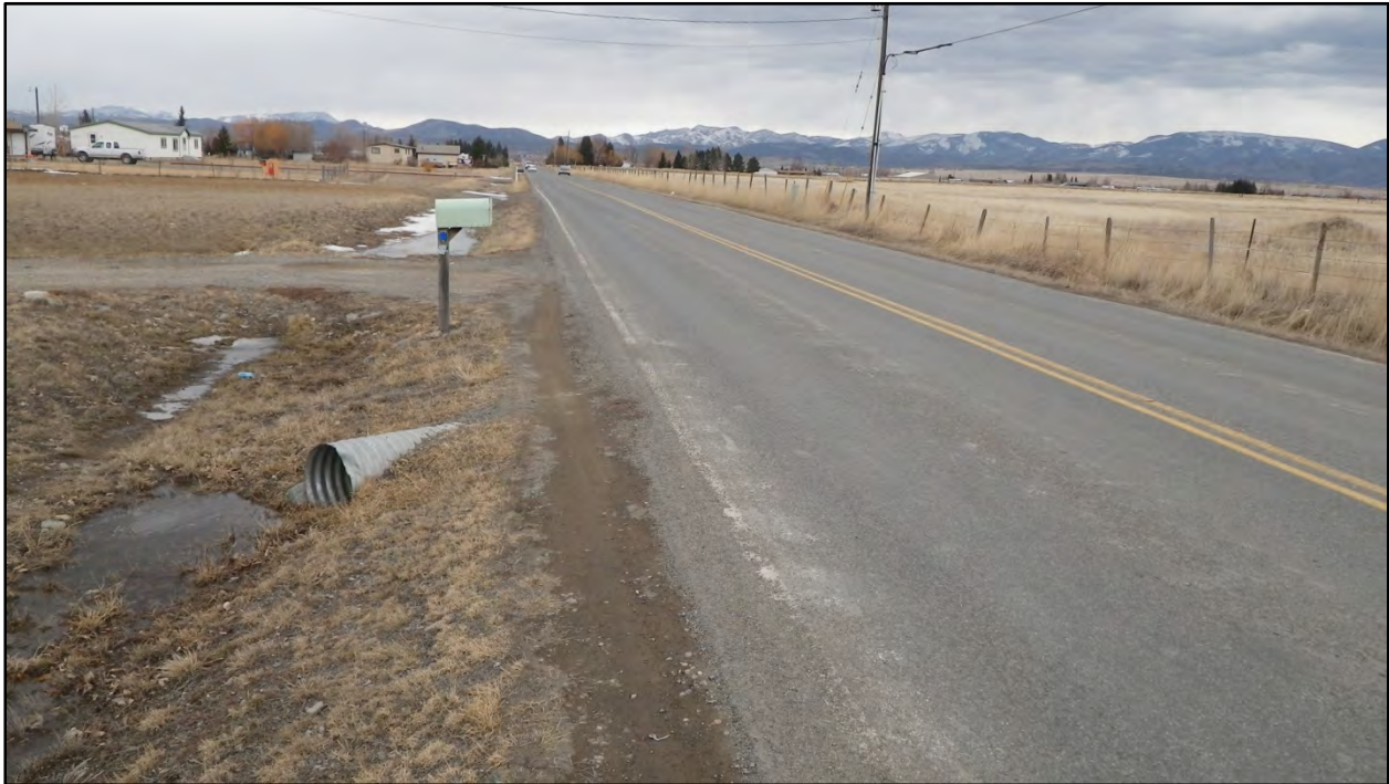
Photo 4.1: Existing cross drain located at MP 1.02.
