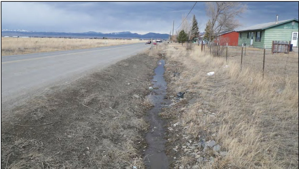
Photo 3.1: Existing Typical Section E.1 looking north.
