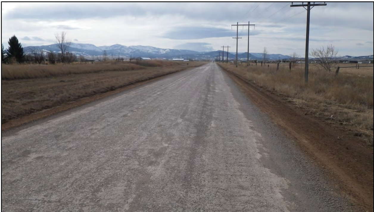
Photo 3.3: Existing Typical Section E.3 looking south.
