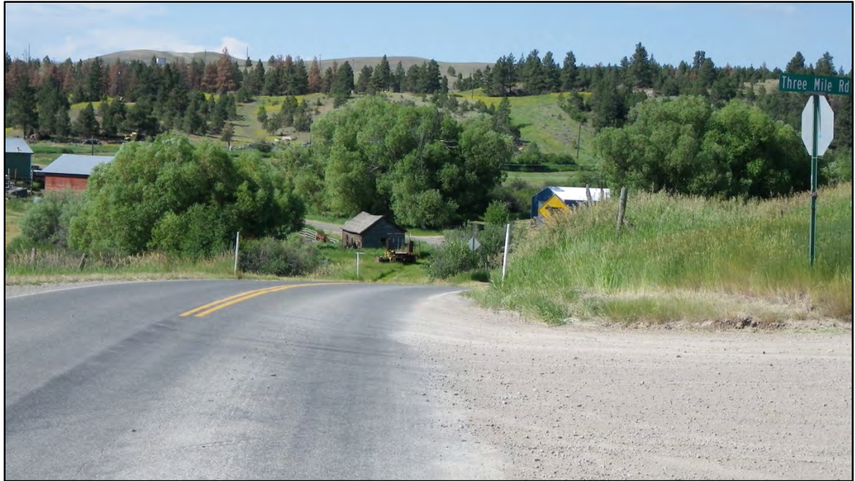
Photo 3.6: Poor sight distance at Three Mile Road intersection near MP 6.55 – Looking Southwest.
