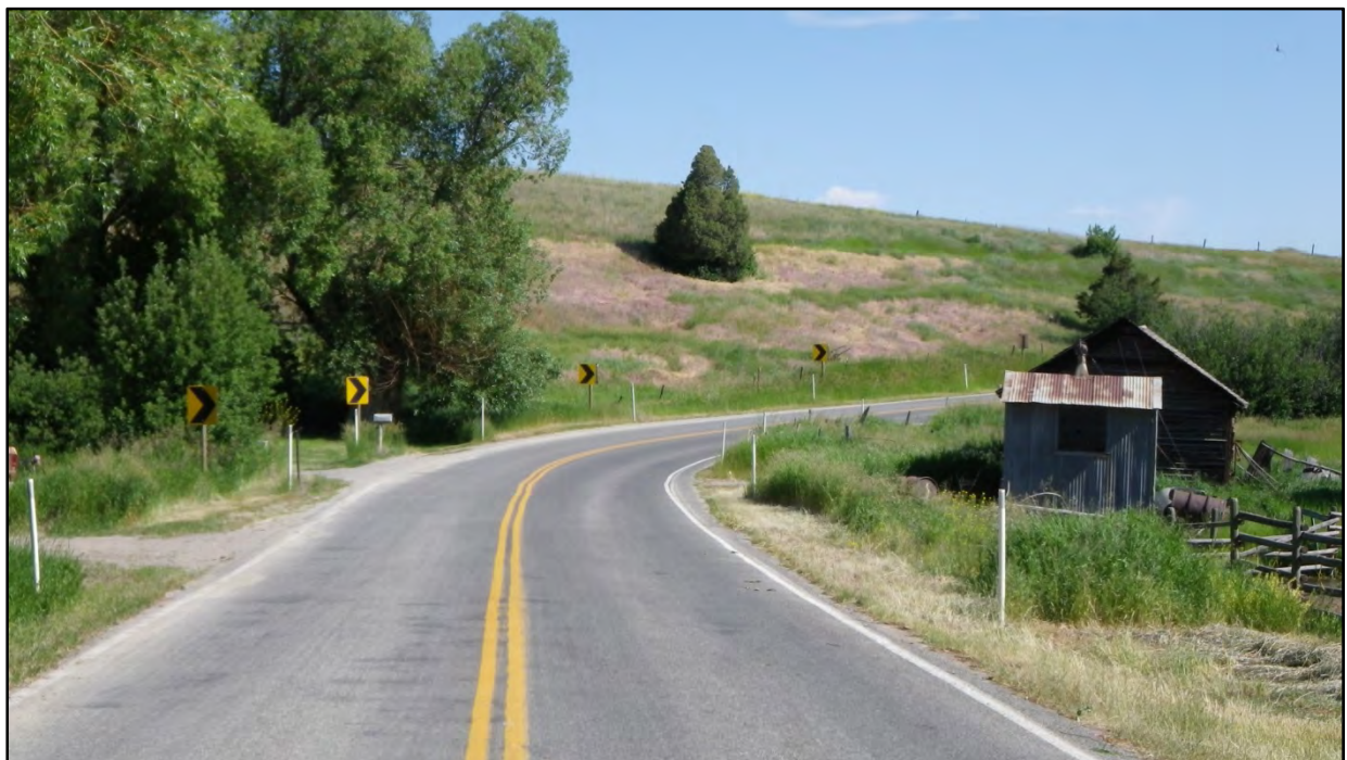
Photo 3.2: Curve and poor sight distance at MP 6.45 – Looking North.
