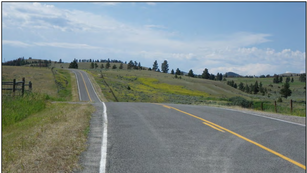
Photo 3.7: Poor sight distance at Hickory Road intersection near MP 7.30 – Looking South.
