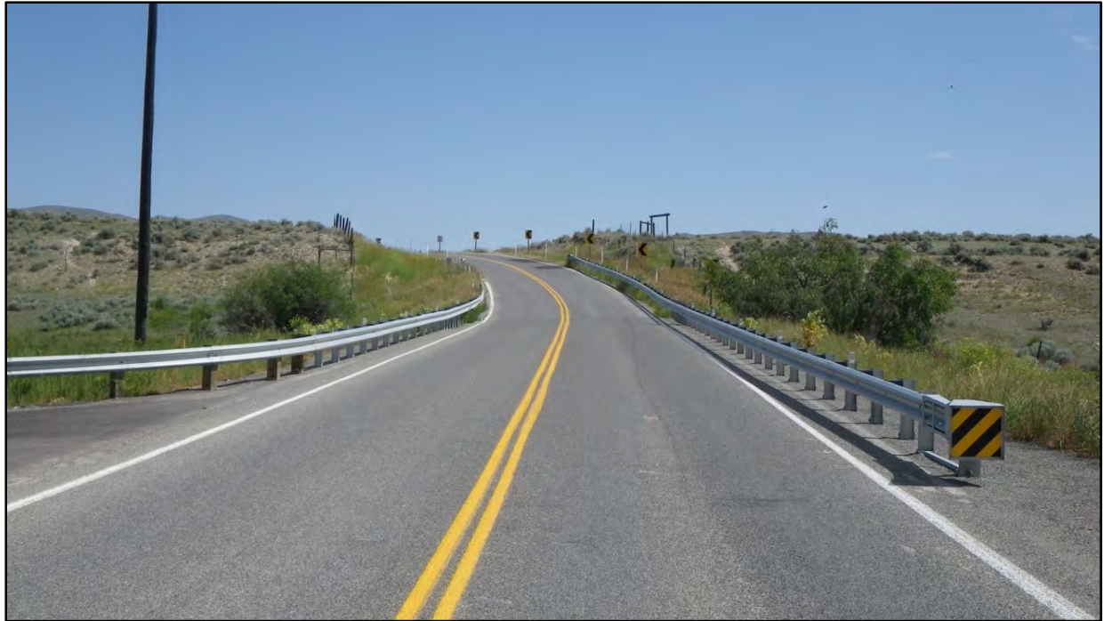
Photo 3.3: End of MDT Safety Improvement Project STPHS-HSIP 25(52) – Looking North.
