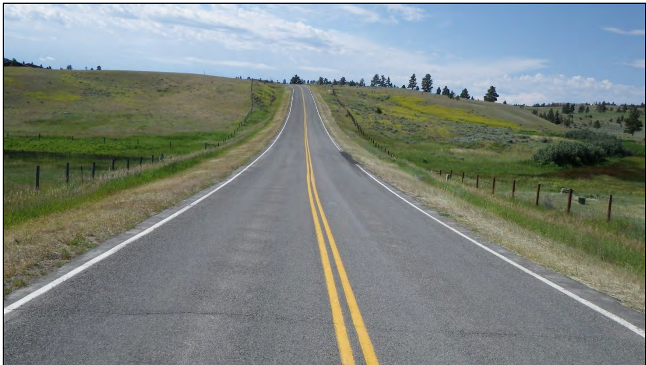
Photo 3.10: Existing Typical Section E.2 – Looking South.
