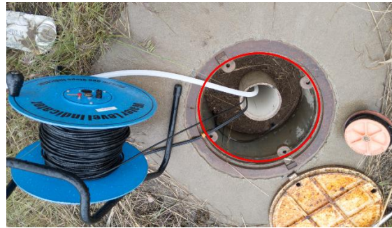
Figure 8: Wells that terminate flush with the ground surface (flush mount) are measured from the steel collar built into the concrete (red circle).
